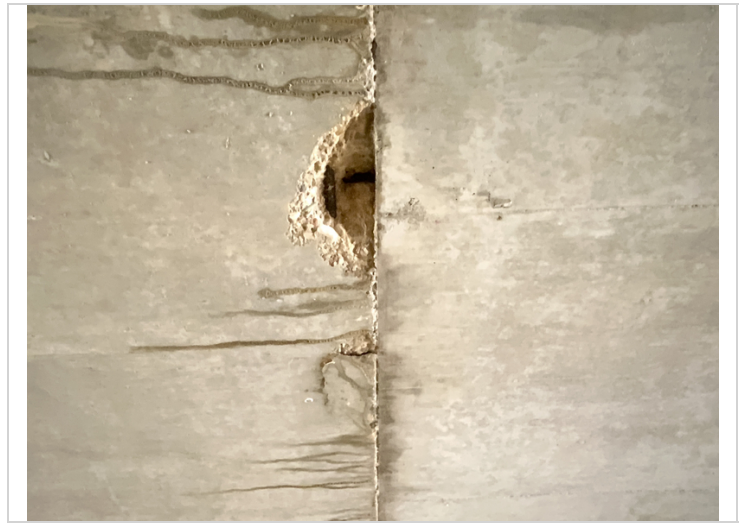
Span 7 at centerline spall with exposed rebar
