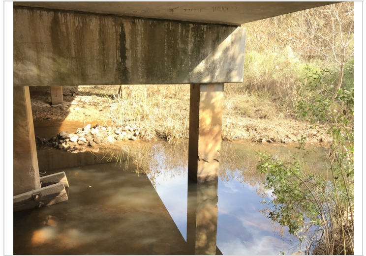
Bent 2 pile 8 appears to have a patch on the back side of the pile from bottom of the cap down about 5';, this was likely a build up on this pile.
