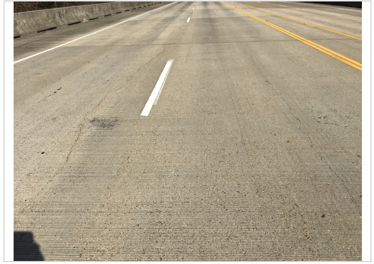
Deck cracks
