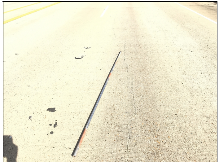
Span 1 longitudinal deck crack, this crack goes full length of the bridge.
