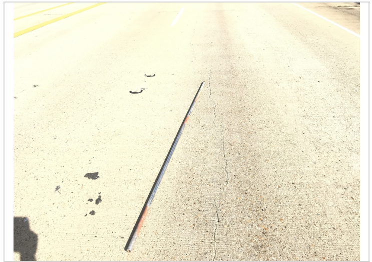
Span 1 longitudinal deck crack, this crack goes full length of the bridge.
