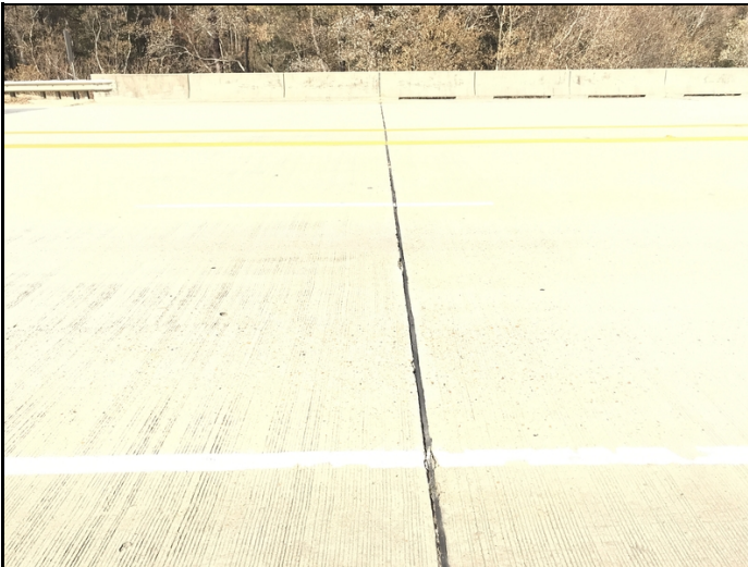
Joint between Spans 1 & 2, joint material is losing bond with the concrete.
