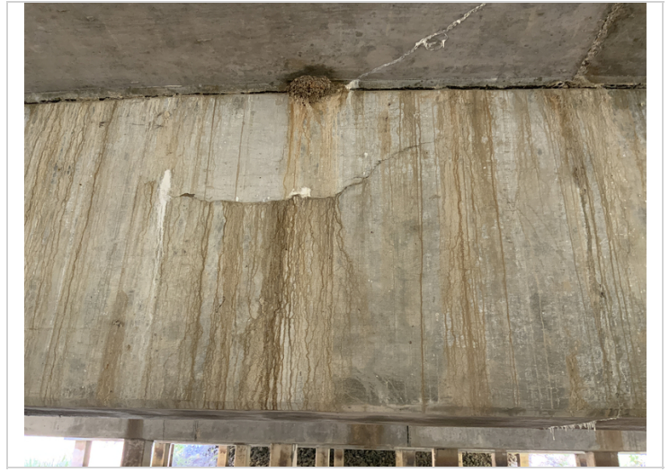
Bent 4 cap, back crack
