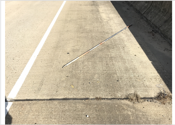
Span 7 Rt. Shoulder diagonal shear crack in deck.
