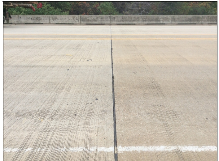
Bent 4 joint material, worn & tattered and losing the bond with the concrete, typical of all joints.
