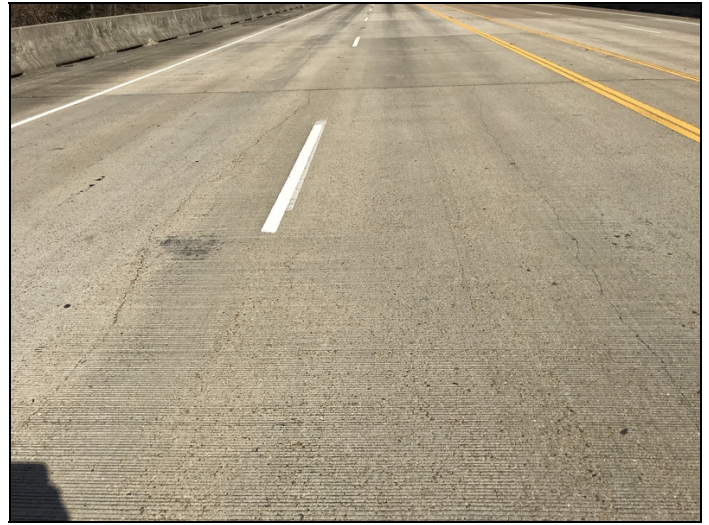
Deck cracks
