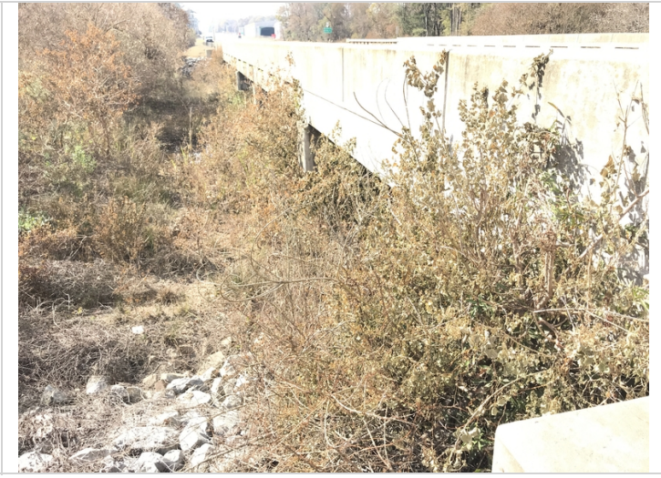
Rt. Side lookingback from abutment 2 @ vegetation growing back under & up beside the bridge.
