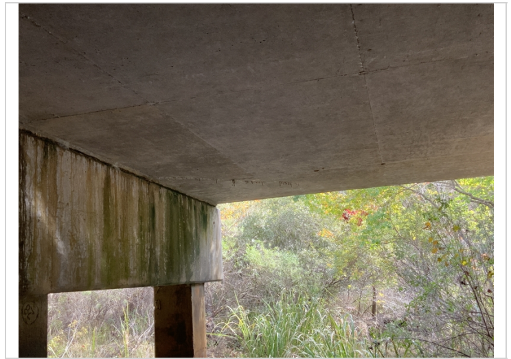
Span 1 efflorescence
