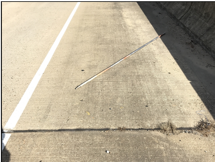
Span 7 Rt. Shoulder diagonal shear crack in deck.
