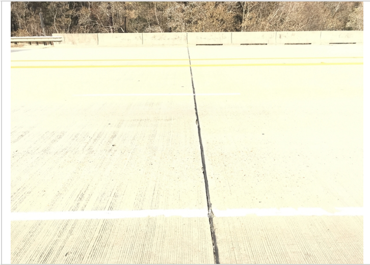
Joint between Spans 1 & 2, joint material is losing bond with the concrete.
